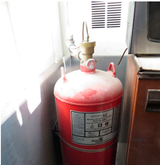
The collision shop's prep booth fire suppression system had not been inspected since 2014.
