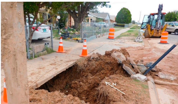
Excavation collapse
