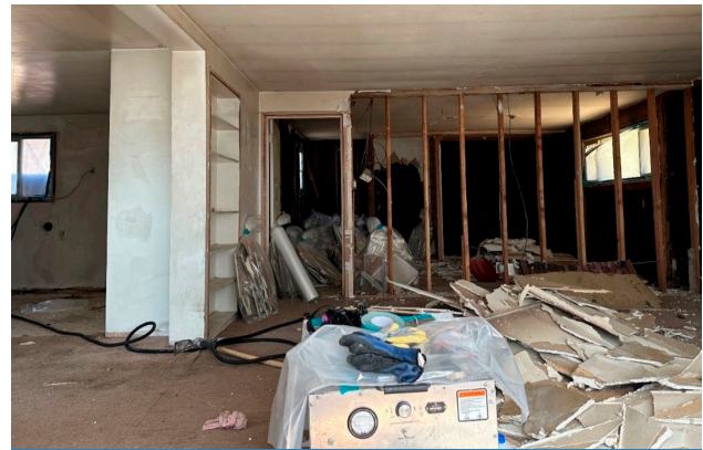
Inside a house where asbestos removal was conducted without following proper procedures.
