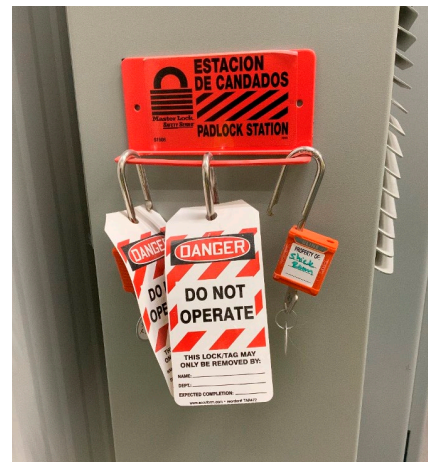
Padlock station with lock/tag.
