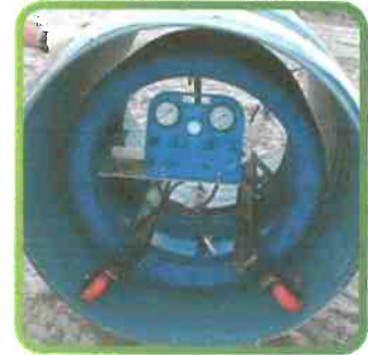
Joint Isolation Test
