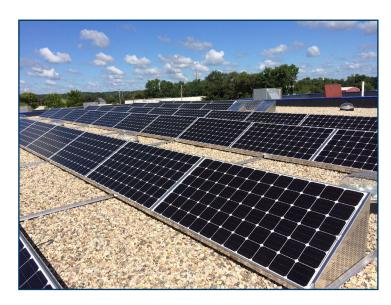
structural engineer. In other buildings, a structural engineer is required to certify that the structural system will provide enough support for the added weight, snow-drift loads and live-load of firefighters.
