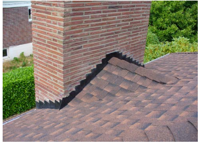
Cricket or saddle at chimney.
