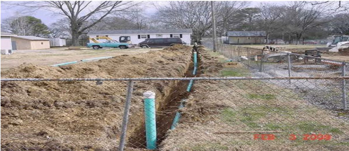
FIGURE 707.4 CLEANOUT REQUIREMENTS
