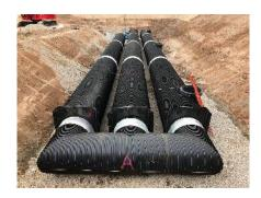
SRPE per ASTM F2562 with internal welded joints under construction at Allianz Field, Saint Paul, MN.
