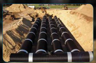
DuroMaxx® Steel Reinforced Polyethylene Technology
