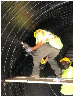
SRPE per ASTM F2562 with internal welded joints under construction at Allianz Field, Saint Paul, MN.
