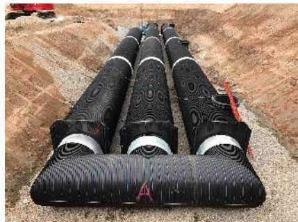
SRPE per ASTM F2562 with internal welded joints under construction at Allianz Field, Saint Paul, MN.
