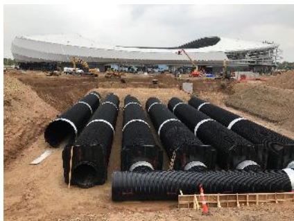
SRPE per ASTM F2562 with internal welded joints under construction at Allianz Field, Saint Paul, MN.
