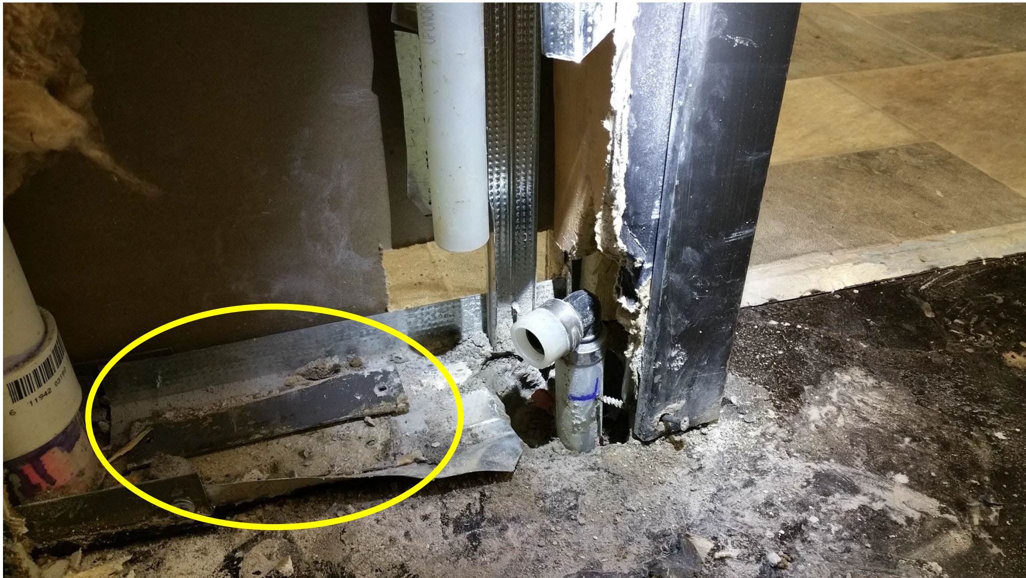
Protection of Piping, Materials, and Structures
