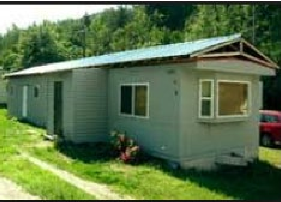
Pre-code non-labeled Constructed Prior to July 1, 1972 ANSI Labeled Structure
