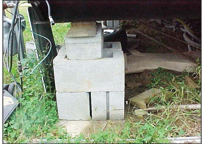
This photo of a non-complying blocking of a manufactured home illustrates why inspections are necessary.
