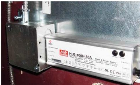
The UL standard restricts the driver output to less than 60 volts in dry applications and less than 30 volts in wet applications. To be listed, the secondary current cannot exceed 5 amps and the total power output rating must be less than 100 watts.
